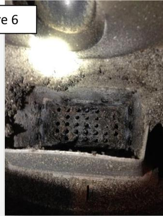
Here is a stove that is well adjusted, even if the ashtray is full fig. 5 the maintenance is well done. There is no black soot on the glass fig. 4 and after burning 6 bags of pellets the burning pot is still clean fig. 6
