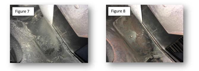
Her is a view from the inside of the smoke chamber in fig 8 you can see the chrome intake of the pressure switch in a Sabrina it is located on the right hand side wall you need to make sure to clean this inlet properly or you will end up whit default start alarm **on a P96x.. it's on the rear wall**
