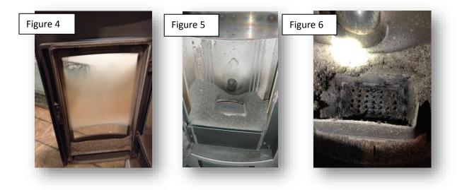
Here is a stove that is well adjusted, even if the ashtray is full fig. 5 the maintenance is well done. There is no black soot on the glass fig. 4 and after burning 6 bags of pellets the burning pot is still clean fig. 6
