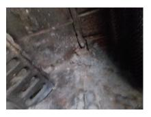
There are cracks evident where the face of the fireplace meets the firebox. These cracks have the potential hazard of allowing heat, sparks and other byproducts of combustion to travel behind the facing material of the fireplace and possibly cause a structural fire. 2016 NFPA 211 11.2.1.5
