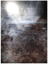
The floor of the firebox has cracks in the mortar and / or bricks or the bricks are pitted. The floor of the firebox needs repaired.
