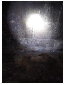
There are gaps in the mortar joints. The smallest gap in the masonry can create a pathway for rogue flue gases to be drawn into areas of the structure that could pose a potential fire or carbon monoxide threat. Fireboxes are to be laid with refractory mortar that can withstand heat and moisture. 2016 NFPA 211 11.2.1.4 IRC 2006 2111.5
