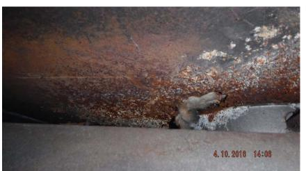
Fireplace is rusted out around damper, recommend not using, potential hazard
