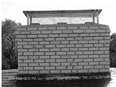
Metal Cap on Clay Liner Chimney Top
