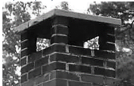
Concrete Cap Chimney Top
