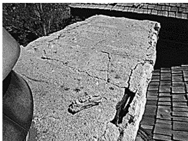
Damaged Chimney Cap
