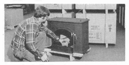
At the final station on the assembly line all warning labels are properly attached and each stove is supplied with manuals, stove legs and accessories. When the stove is then ready, it is boxed and prepared for shipment. The stoves are then mounted on sturdily-built wooden skids. Upland goes to this expense because it assures us of a perfect stove reaching the customer.
