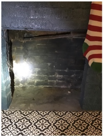
Firebox deteriorated
