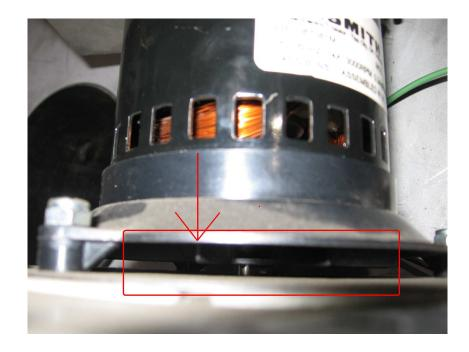
4- Insert a screw driver between the motor and the fan to separate the venting fins from the venting assembly by about ¼ in
