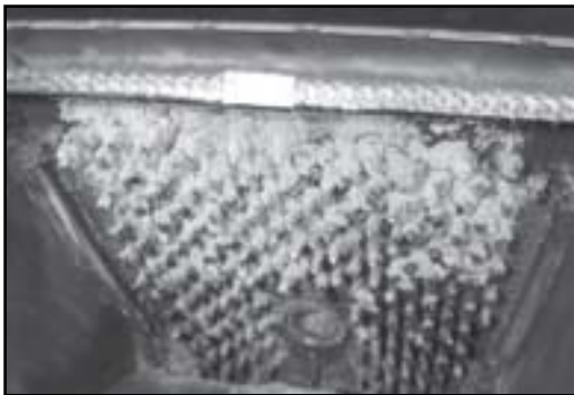
Figure 1 - Example of a dirty heat exchanger
