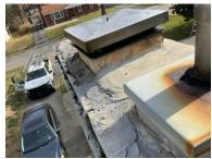
The crown / wash cap of the chimney is not constructed in a way that properly protects the chimney. The crown should be constructed with concrete. It must have an expansion joint around the flue tile. It should overhang the main structure to allow a drip edge to protect the chimney. A properly made crown will help protect the chimney from water intrusion and damage.
