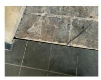
There is a gap between the hearth and hearth extension. Sparks and embers can fall through the crack posing a potential risk.
