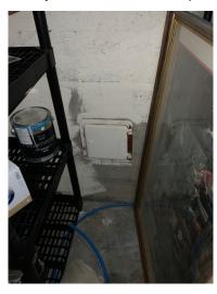
There are combustible materials that are too close to the ash cleanout door. This could potentially be a fire hazard. The Clearance to combustibles is to be 18" 2016 NFPA 211 7.1.4.5 IRC 2006
