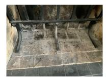
The firebox has deteriorated mortar joints. Firebrick are to be laid with a medium-duty refractory mortar. The with of the joints in the firebox should not exceed 1/4". 2016 NFPA 211 11.2.1.4 IRC 2006 2111.5
