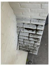
There is significant deterioration in the mortar between the bricks. This can not only allow water intrusion into the chimney and cause potential leaks inside the home, but it also allows water into the chimney which can damage the chimney structure.
