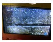
The flue is coated in creosote and soot. This could be the fuel that would lead to a flue fire. 2016 NFPA 211 7.2.13.3
