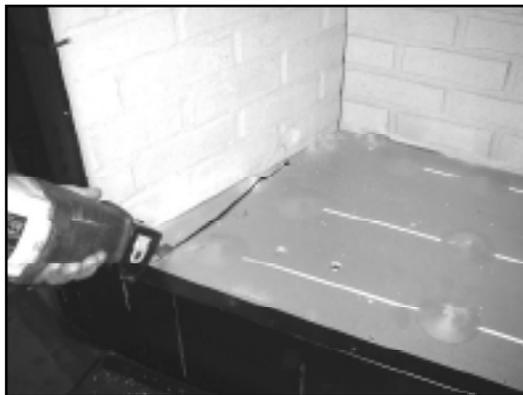
**Figure 11.2.** Using a saws-all, cut out the floor.
