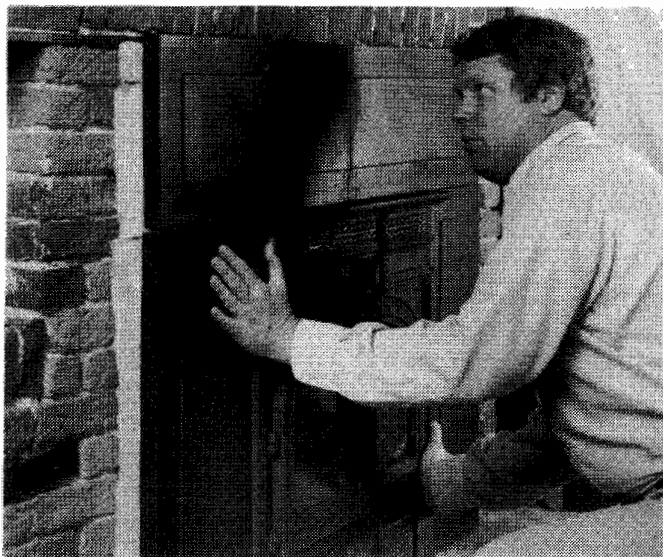
COMPRESSING THE INSULATION TO THE FIREPLACE FACE
